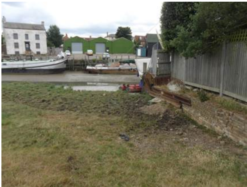
Photograph 1.2 – Location L, again the ramp rises to match the existing wall.
